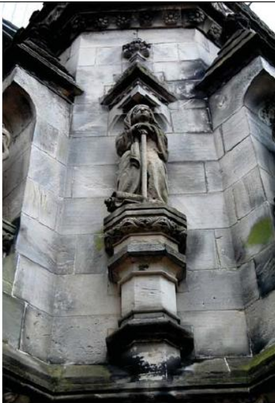
External detail from the Victorian baptistry
